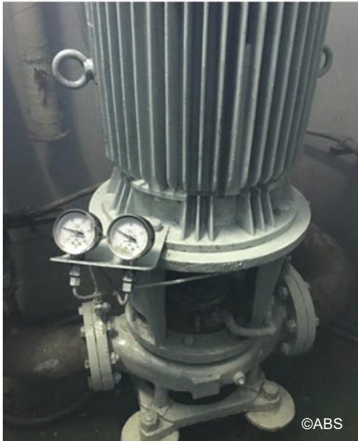
Fire pump running after repairs
