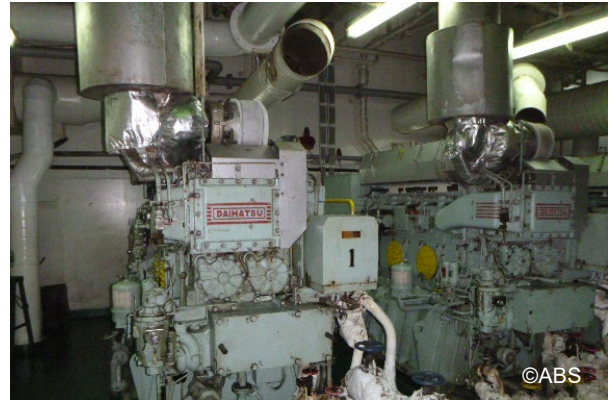
Auxiliary engine exhaust insulation renewed
