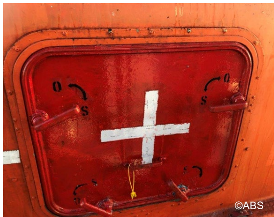
Lifeboat door not closing properly – after repair
